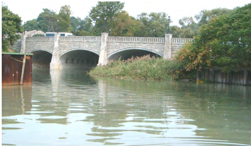
Overpass near Mill Pond weir (CSHH #13) (photo by Carol DiPaolo)
