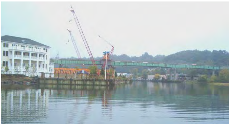
Construction at Roslyn Viaduct (photo by Carol DiPaolo)
